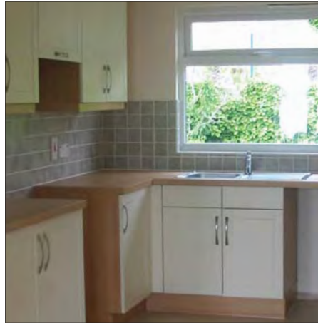
The kitchens at Warren Court have been upgraded as part of the refurbishment.
