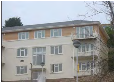
An extra storey has been created at Warren Court.
