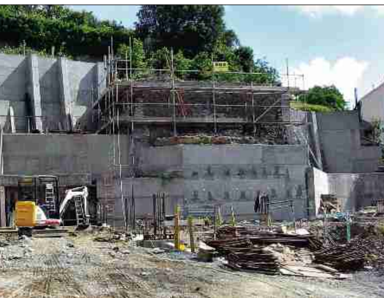
The rear of the site is being stabilised
