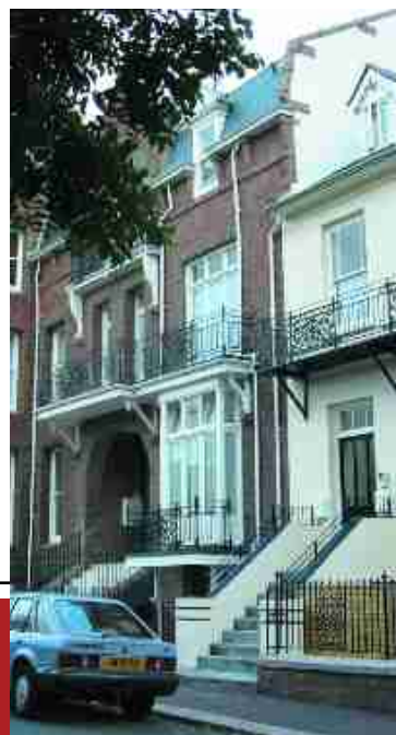
The original façade of the former hotel and several other features of the building have been retained at Parkside
