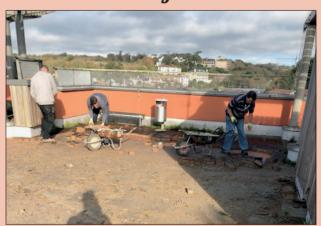
Work is continuing to re-surface the roof garden at Le Coie in Springfield Road. Since the development opened in 2006 there have been problems with water leaking to communal areas below.
